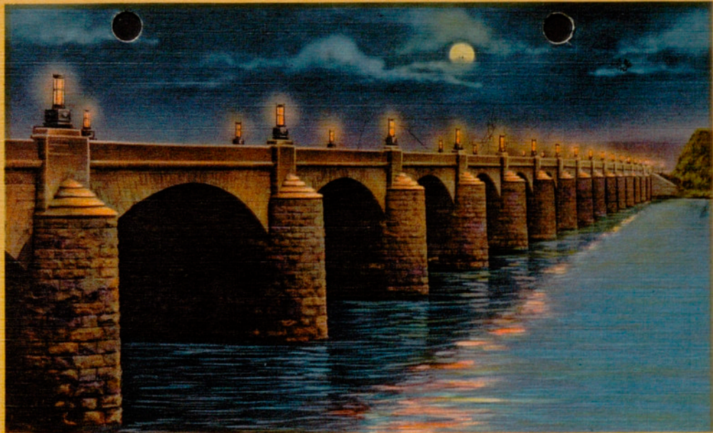
3—Market Street Bridge at Night, one of Pennsylvania's Finest Bridges, Harrisburg, Pa.
